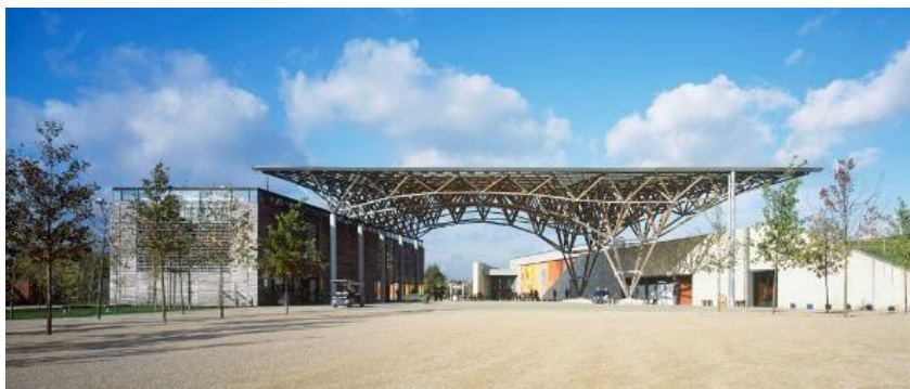
Figure 6 : Earth Canopy, designed by Feilden Clegg and Atelier One (Atelier One 2015)
